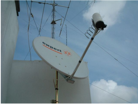
Photo n°2: Solid aluminium offset fed dish
